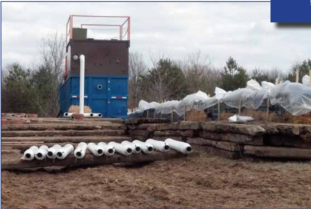
Water Matrix setup next to pond #1 with first bank of Floc Hogs.
