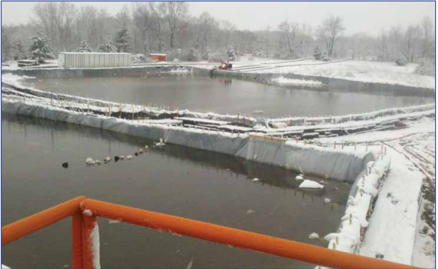
View of ponds from the top of container based water treatment and clarification system.
