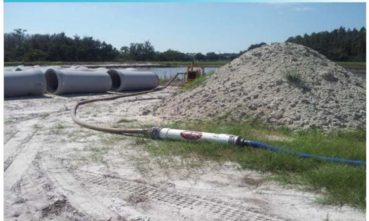
Floc Hog connected to 4" lay flat hose
